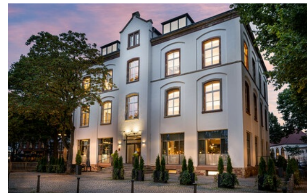
Member Relais & Châteaux since 2023 Nauwieserstraße 5 66111, Saarbrücken
